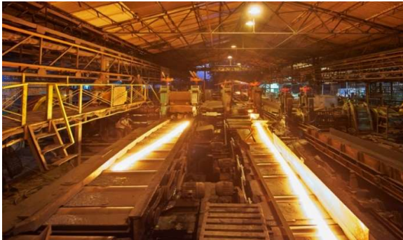
Structural Steel Rolling Mill
